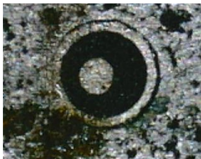
Figure 3-21: Conductivity pin as seen from pipe inside (courtesy Al Schubert).
